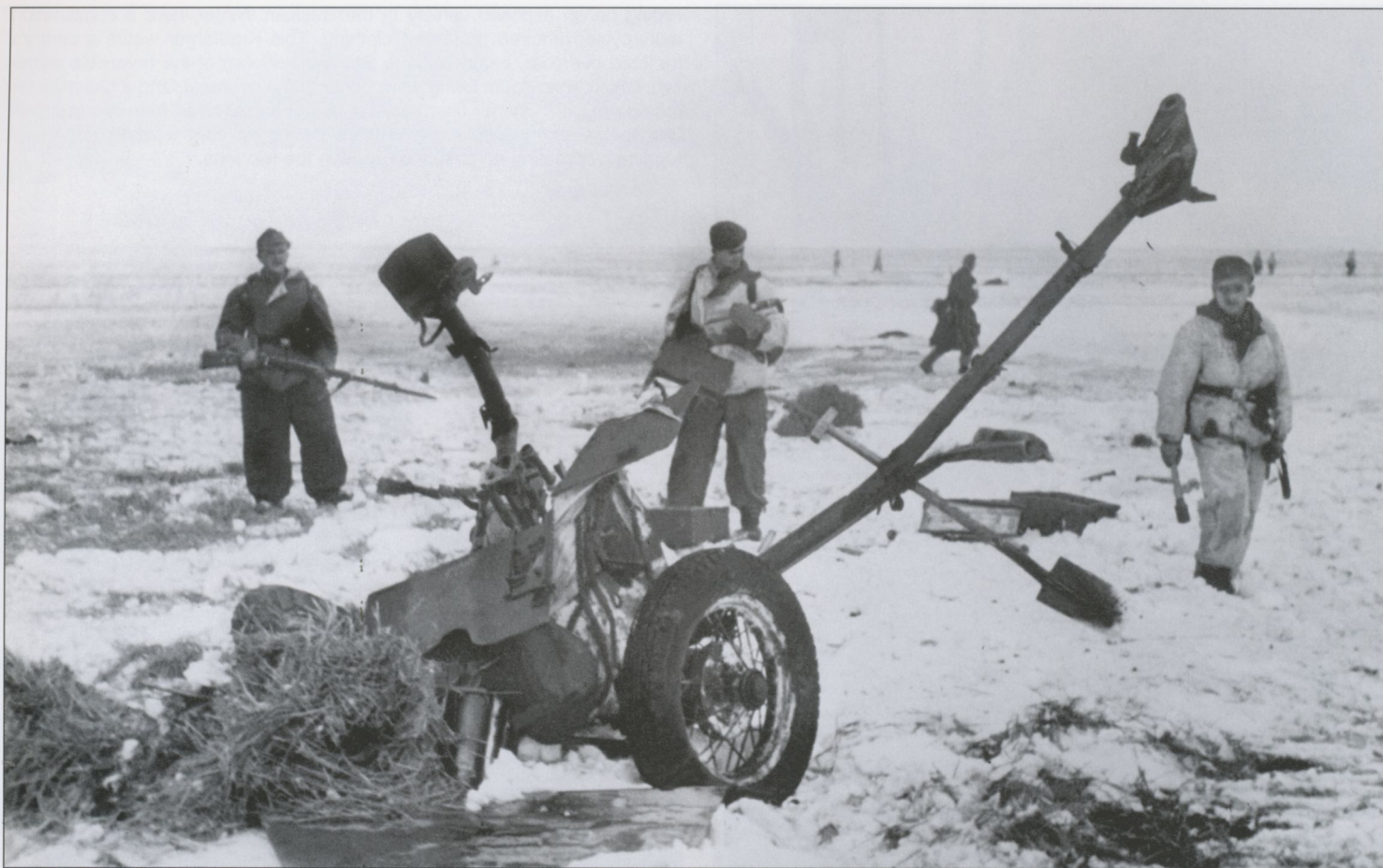
Advancing German troops inspect a damaged Soviet 45mm M1937 or M1942 (longer barrel) antitank gun. These were licensed copies of the 3.7cm PaK35/36 and were first produced as the 37mm M1930 and M1932. They were re-barreled to 45mm so they could fire a more effective high explosive round. The Soviets desired their weapons to be more multi-purpose. The Germans captured large numbers in 1941-42 and pressed them into service as the 4.5cm PaK184(r) and PaK184/1(r).
