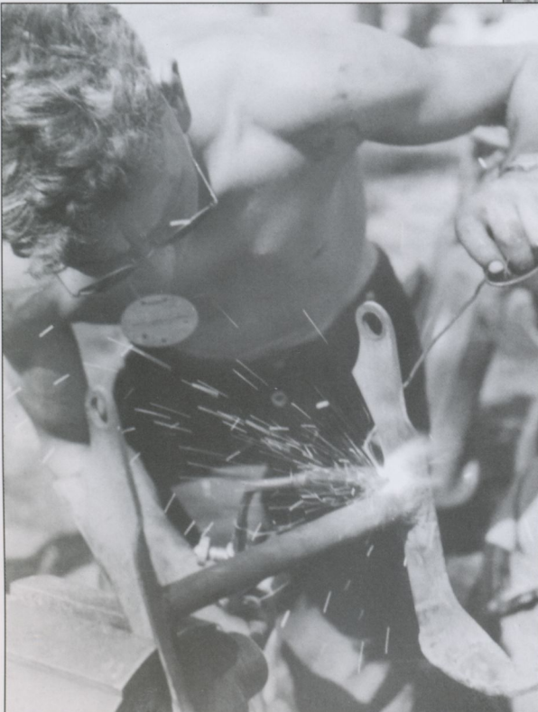
An artificer brazes a damaged vehicle part with a blowtorch. Note this sunglasses used for eye protection. His identity tag (Erkennungsmarke) is worn around his neck. Both halves bore the individual's unit designation, unit roster number, and blood group. If killed the bottom half of the tag was broken off and turned into the unit and the other remained with the body. The Landser referred to it as a Hundemarke (dog tag).
