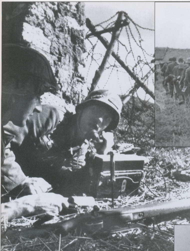
A Leutnant reports the situation to his higher headquarters via a field telephone 33 (Feldfernsprecher 33). This set weighed 12 pounds. It operates on the ground-return principal. Instead of two wires, only a single-wire line was used. Between the telephone and the carbine can be seen a rod with a grip handle stuck in the ground and connected to the telephone by a short wire. This took the place of the second wire. Damp ground improved transmission range.
