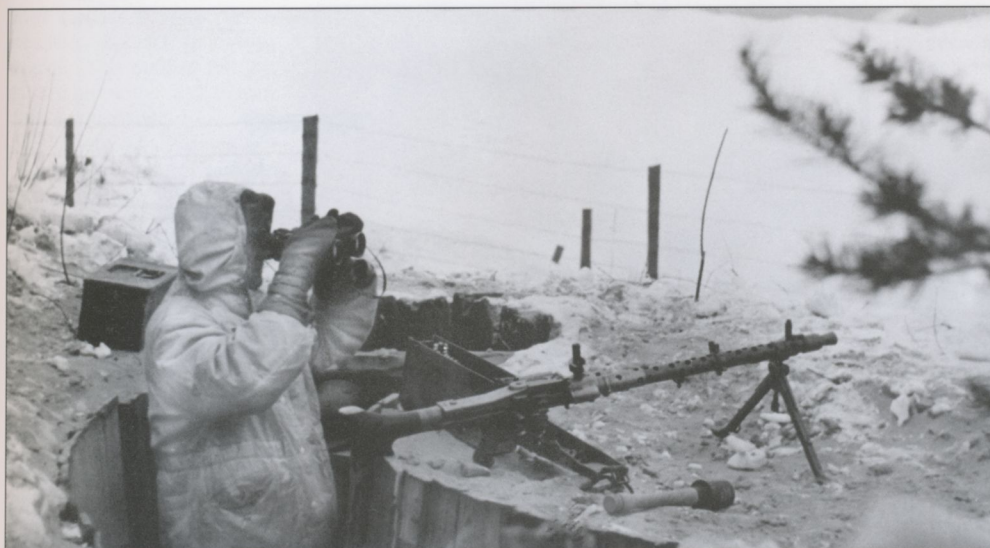
This MG34 light machine gun position (Schützenloch für leichtes Maschinengewehr) is revetted by vertical planks. Small one-man dugouts are located at both ends of the position. On the forward side was a 20cm deep U-shaped platform for the bipod-mounted gun. Spoil was removed to hide the position.
